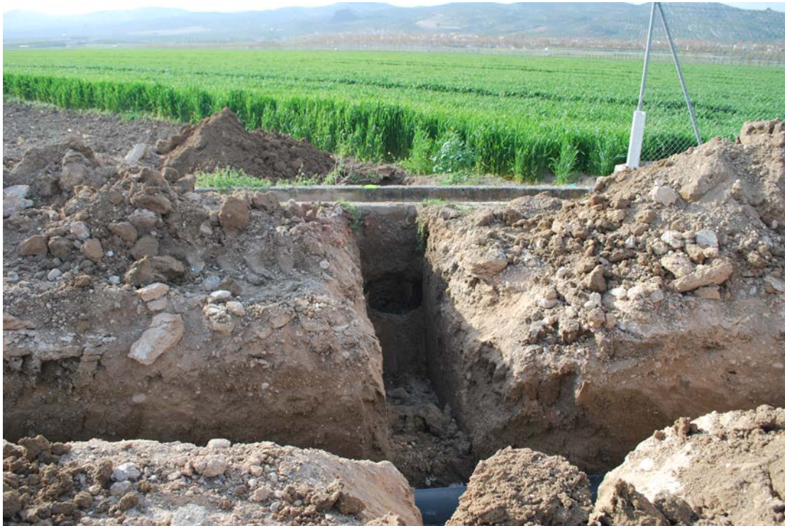
Modernization works of a HIS through the replacement of open channels by an underground pipe distribution network
